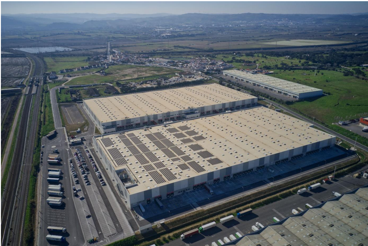
© Aquila Capital – Rainha Green Logistics Park (Azambuja, Portugal)
